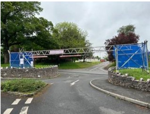
Kirkby Stephen Town Council Temporary Barrier Works.
